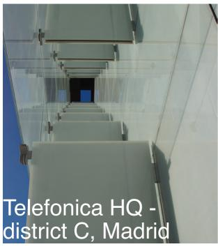
The media center of the Northern Madrid Telephone Company includes 12 office buildings. Prominent components of the complex are floating roofs and a double envelope made of light louvers for wind orientation and avoiding direct sunlight radiation. Internal selective insulated panels enable the penetration of filtered light into internal spaces, improving functional efficiency in accordance with strict green building standards.
