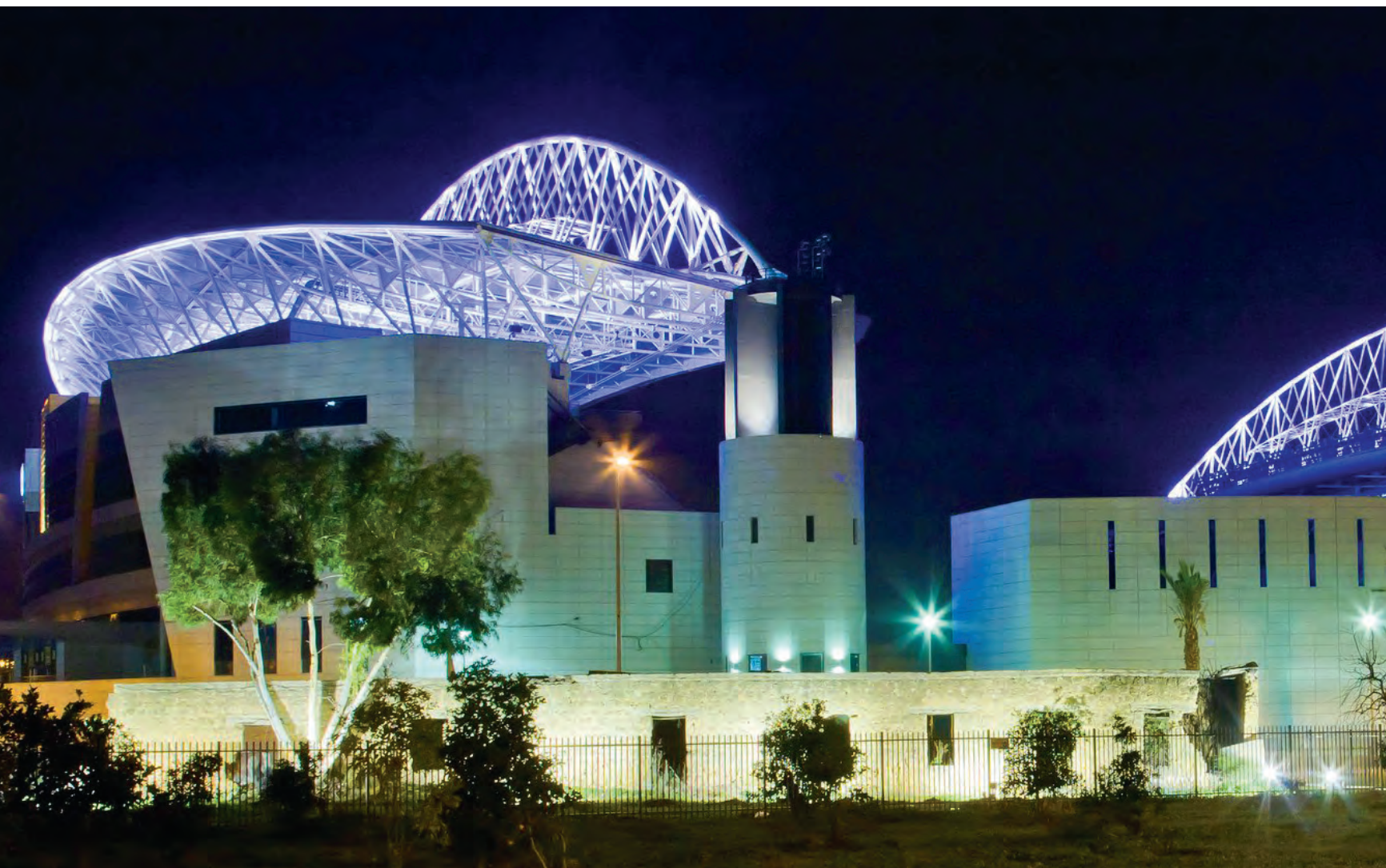
Top: South-west view of the Netanya stadium. Bottom: Aerial view with site plan on the right. Goldshmidt Arddity Ben Nayim Architects
