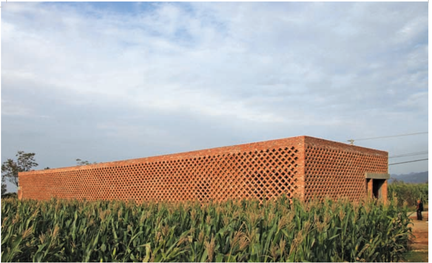
Ecological house for all seasons, China Open and closed spaces defined by the inhabitants with self-made mud bricks behind the homogenous industrial brick wall, expressing the family's needs around the year.
